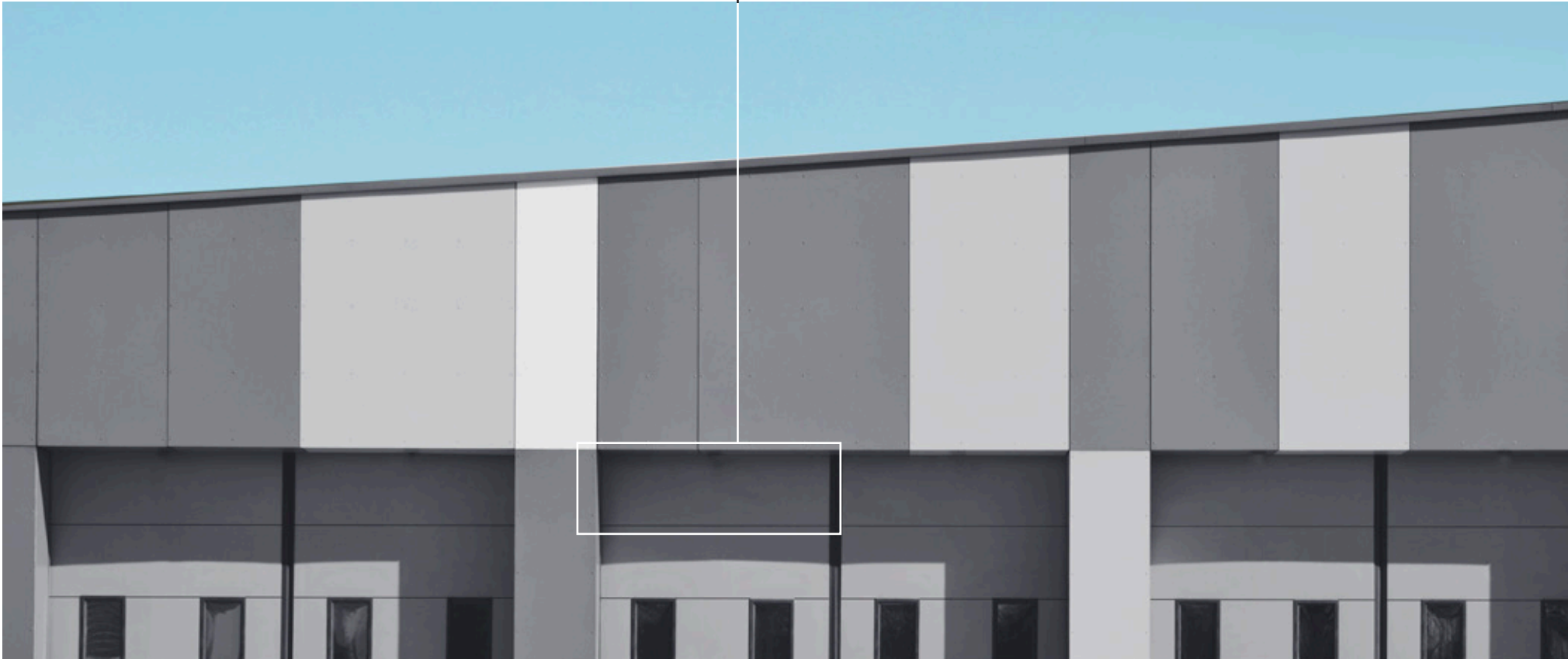
Dummy modules used to cover the shaded parts.
